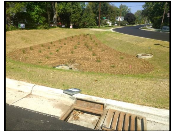
Structure located upstream of infiltration basin
